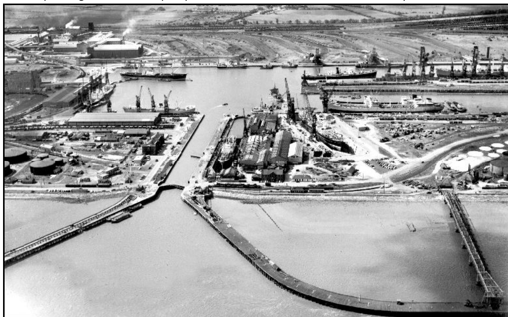
These aerial views show the new Henderson Graving Dock. In the upper view it is empty. In the lower view a vessel is receiving attention. The coal hoist on the Western Jetty has gone and the rail bridge replaced by a pipeline, the jetty now serving as an oil terminal. The photo gives a similar perspective as the souvenir edition's 'Bird-Eye View'. both IMM
