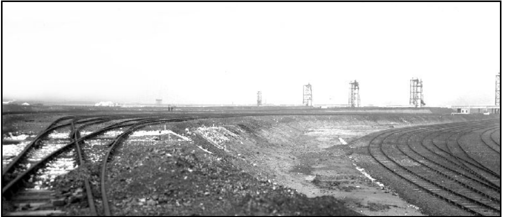
▲ The expanse of sidings constructed to supply the coal hoists in the distance. IMM ▼ The seven coal hoists along the south quay of the dock look ready for action although the quay in the foreground still needs some work doing on it. IMM
