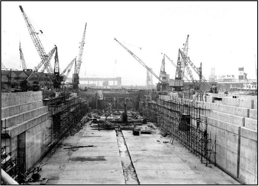
A larger graving dock was opened on 21 Oct. 1960 and was named the Henderson Graving Dock. It was located to the west of the old graving dock. This allowed larger vessels to undergo repair at Immingham. The upper view shows the dock under construction and the lower view shows the dock filled with water. The entrance to the dock was adjacent to the old graving dock entrance. both IMM
