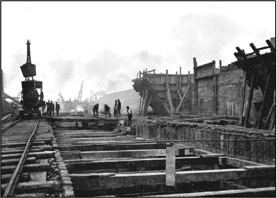
Work progressing on what looks like the entrance lock.
