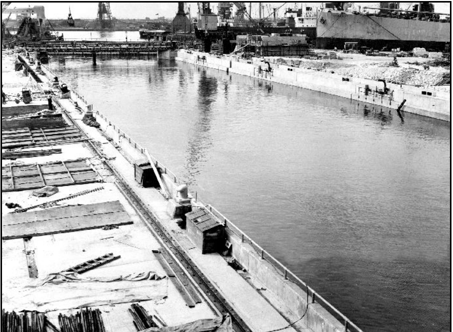
A larger graving dock was opened on 21 Oct. 1960 and was named the Henderson Graving Dock. It was located to the west of the old graving dock. This allowed larger vessels to undergo repair at Immingham. The upper view shows the dock under construction and the lower view shows the dock filled with water. The entrance to the dock was adjacent to the old graving dock entrance. both IMM
