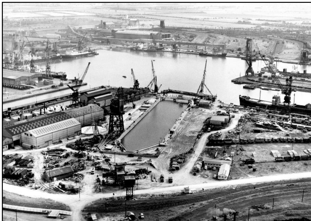
These aerial views show the new Henderson Graving Dock. In the upper view it is empty. In the lower view a vessel is receiving attention. The coal hoist on the Western Jetty has gone and the rail bridge replaced by a pipeline, the jetty now serving as an oil terminal. The photo gives a similar perspective as the souvenir edition's 'Bird-Eye View'. both IMM
