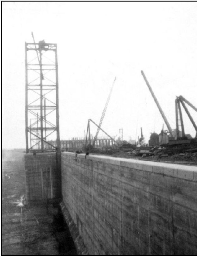
A coal hoist under construction. Seven of these were placed along the south side of the south western arm. IMM
